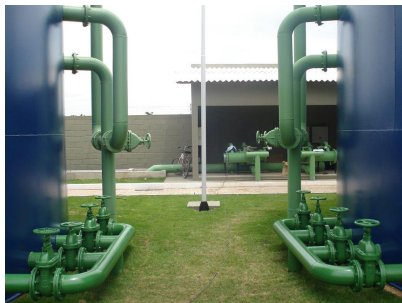
ETE ULISSES GUIMARÃES BARRILETE
